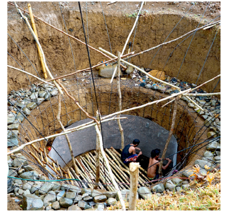
Building a well.
