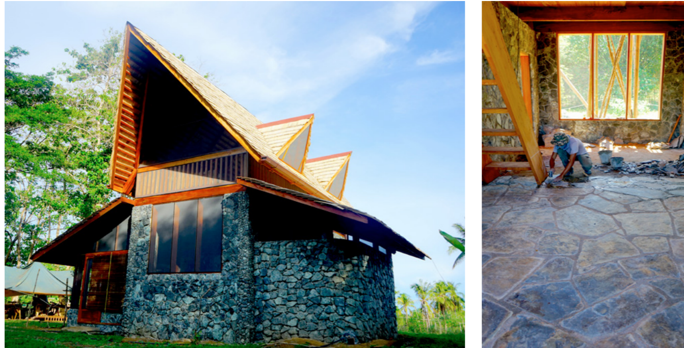
Our first barn house displaying masonry and design features uncommon to Palawan.
