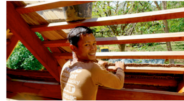
Installing bamboo shingles.
