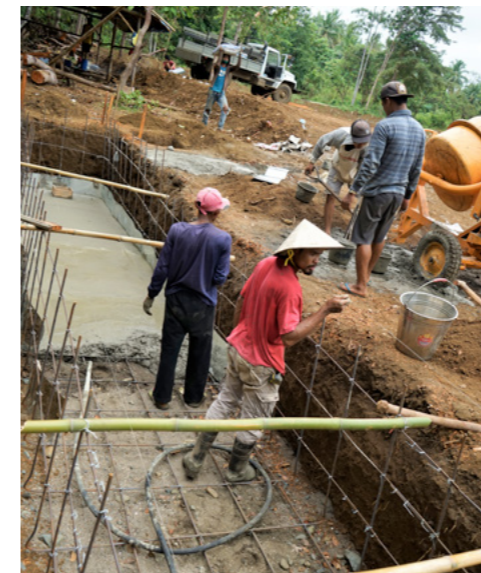
Pouring concrete for the bamboo treatment pool, working to plans designed by our german partners.
